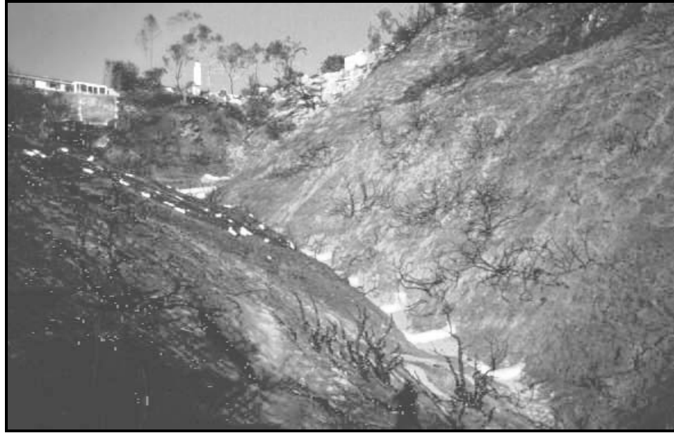
Denuded Slopes Due To Fire
