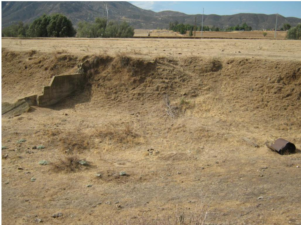
Photograph 21: Dilapidated drainage control structure in Pershing Creek.
