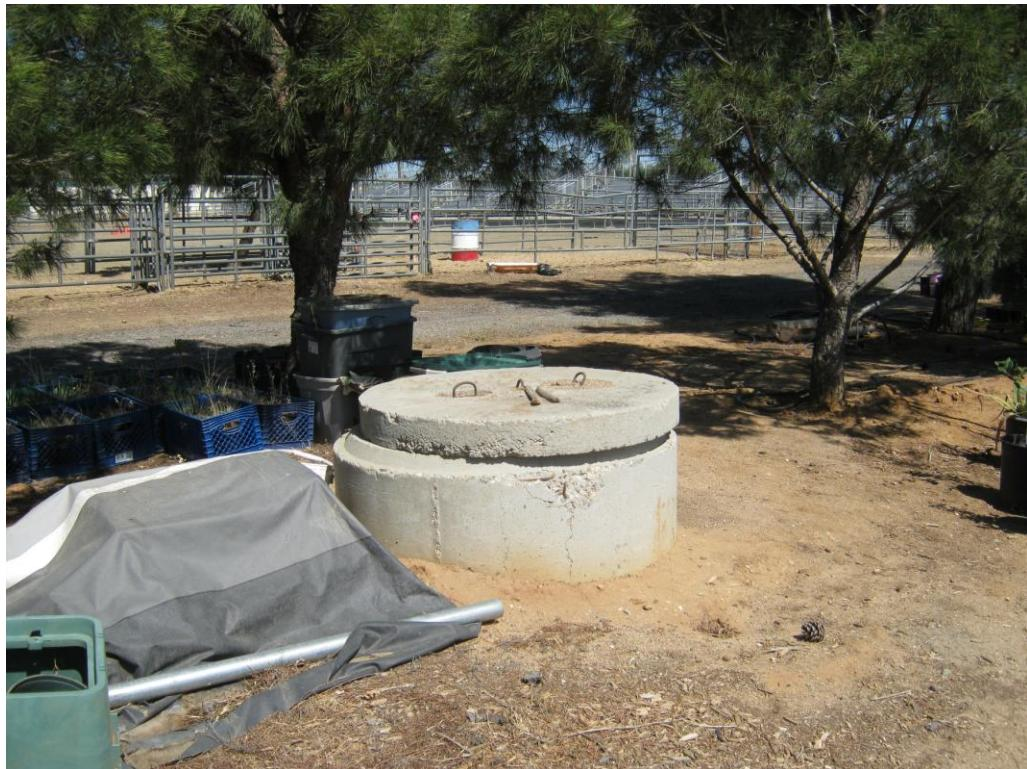
Photograph 10: Concrete standpipe
