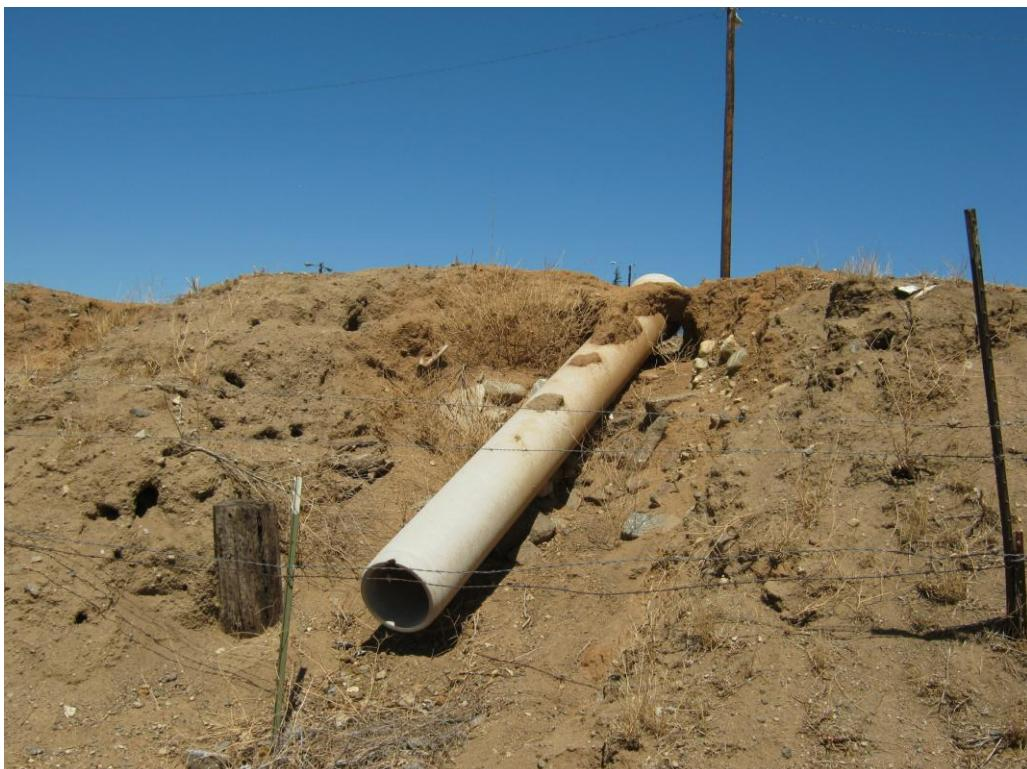
Photograph 4: Transite pipe that directs surface runoff from the equestrian center onto the site.
